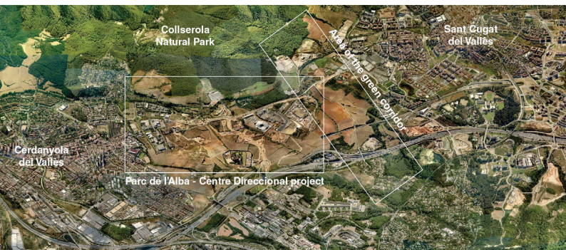
Figure 10 - The area of the green corridor while the project of the Directional Center was under construction
