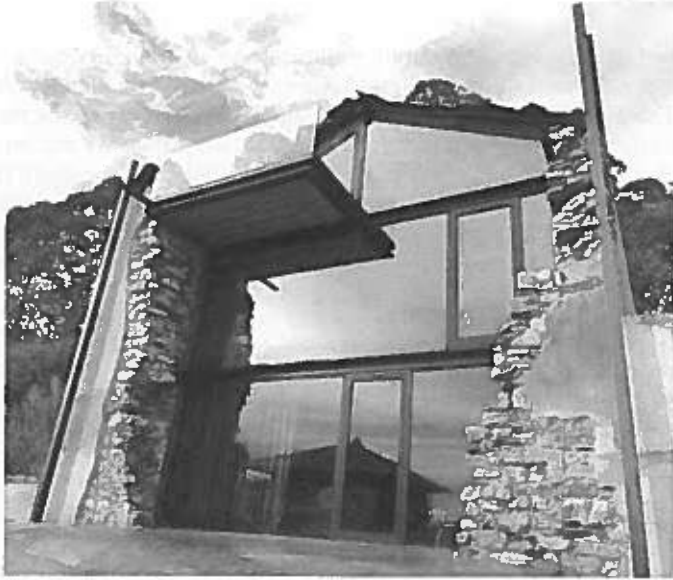
Figure 4. Casa Sabugo, Gijón, Spain (2016), Arch. Tagarro; Arch. De Miguel: Single-family homes restoration.
