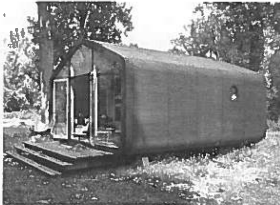
Figure 5. Wickelhouse (2017), developed by the Dutch company fiction factory, Is made out of cardboard, modular and highly customisable, built to last between 50 and 100 years.
